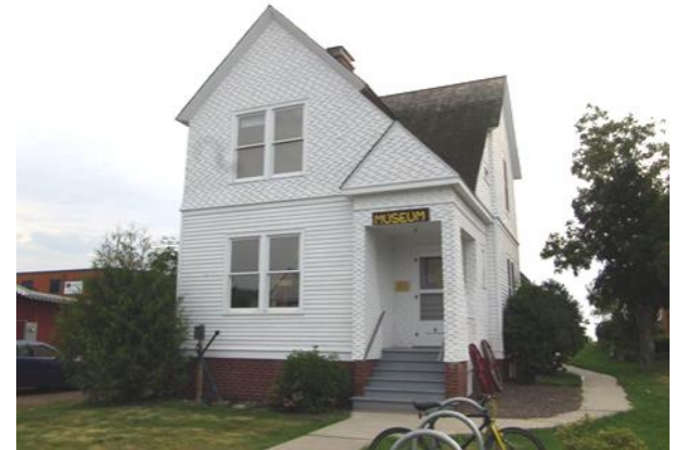
Museum's front entrance (above). Sidewalk was added to the south of the building for handicap accessibility at the back of the building. However, an accessible front entrance needs to be considered for ADA compliance.
